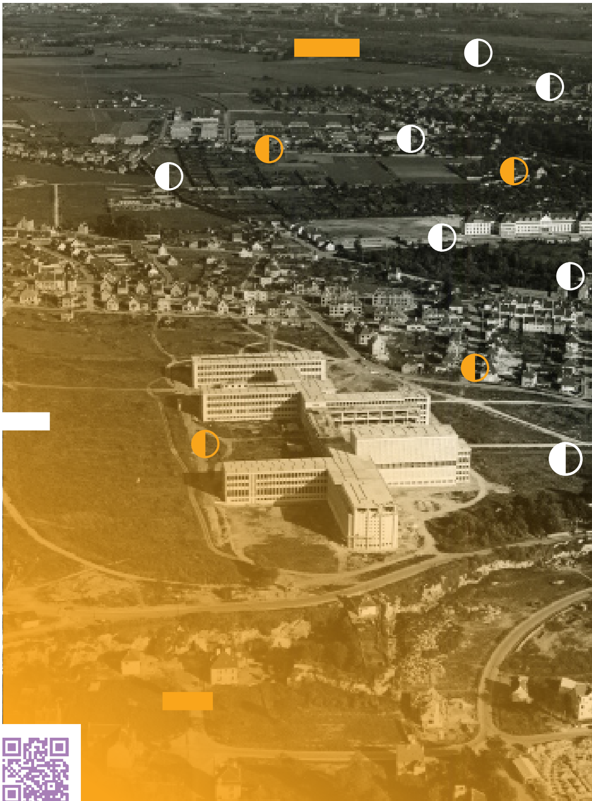
Archival photographs – Construction of the main campus in the 50's
